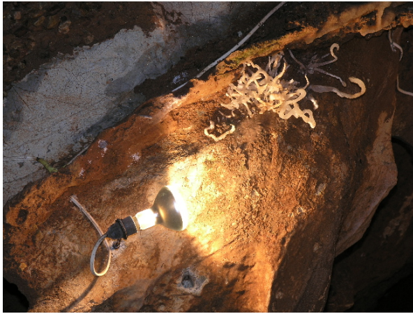
Old light fixture in the Baal showing cabling, drill holes and proximity to fragile crystal
