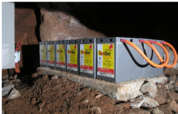
Battery Bank (12 X 2v Sealed gel-cell batteries)
